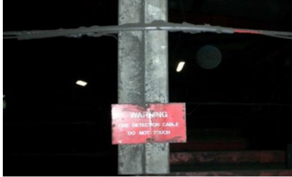
LHDC and Catenary Wire Support
