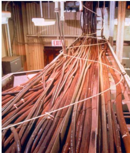
With the monitor modules for the sensor cable, we can be informed of in which meter the incident has occurred. This utility comes in handy in hidden places (skids or false floors) and also in cable galleries for a quick location of the possible fire. In addition, with TASC CTI modules, an alarm can be discriminated from a mechanical short circuit. This feature is unique in heat-melting sensor cables on the market.
