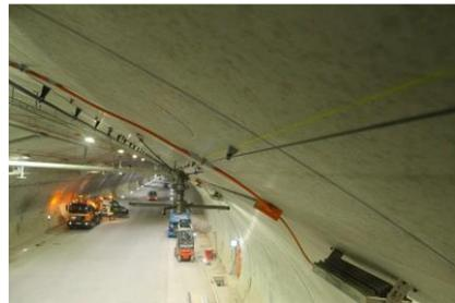
The same cable could also protect galleries of facilities and evacuation routes from tunnels.
